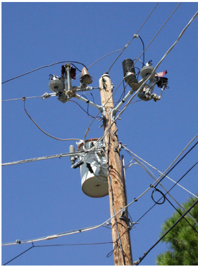
The Cottonwood BPL field trial uses Mitsubishi Electric PLCLINK equipment. [Ernie Cummings, K6XF, Photo]
